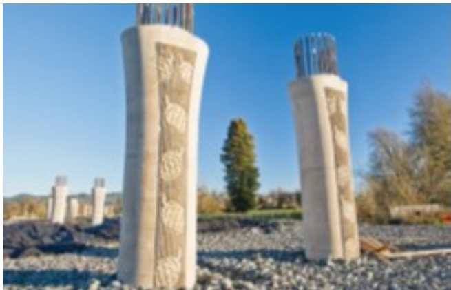
These columns, or bents, rise over 20 feet to support the 1.1 mile viaduct. In all, 64 of these columns support the viaduct's roadway.
