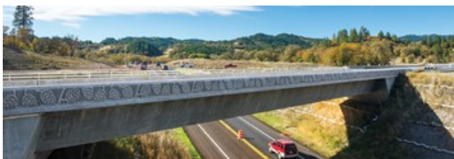
The southbound U.S. Highway 101 bridge spans State Route 20 at the new southern interchange of the Willits Bypass. Note the unique redwood cone pattern designed just for this project. These redwood cones adorn all the concrete structures of the bypass, which opened in November 2016. Caltrans photo by Scott Lorenzo.
